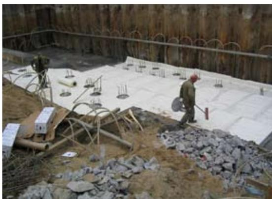
Preprufe being installed below the slab
